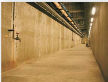
Walls dry after crack injection
