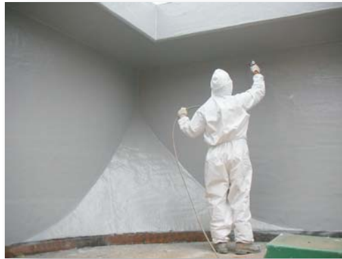
Spray-application of topcoat
