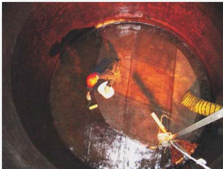
Application of waxcoat - top view
