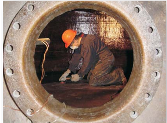
Sanding prior to application of waxcoat
