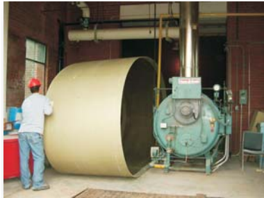
Shell section moved into building
