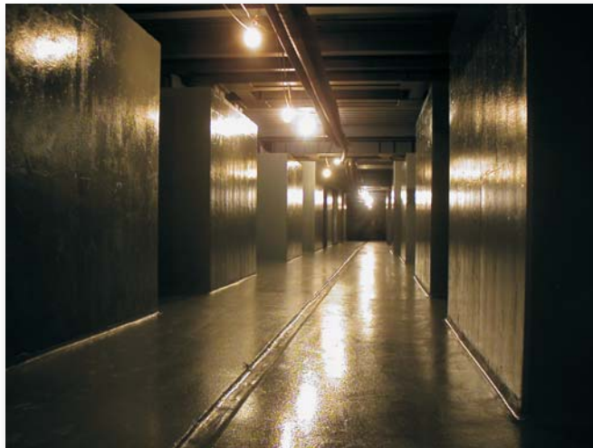
Finished conveyor pit
