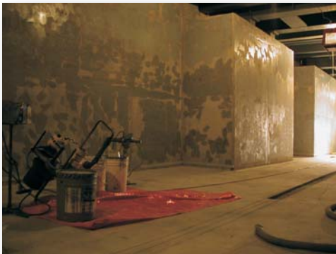
Walls parged prior to coating
