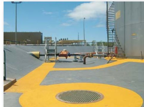
Concrete sump and pedestrian walkway
