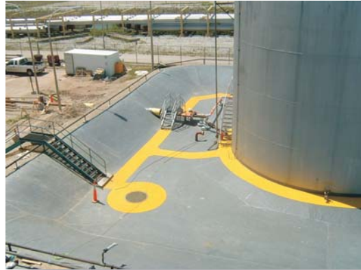
Completed secondary containment membrane
