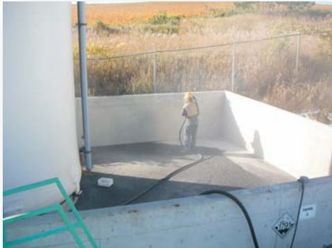
Abrasive blasting preparation of concrete
