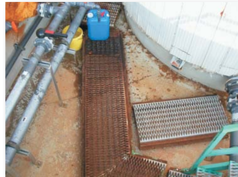
Original condition of containment area
