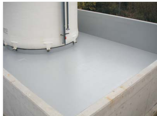
Completed sodium hypochlorite containment area
