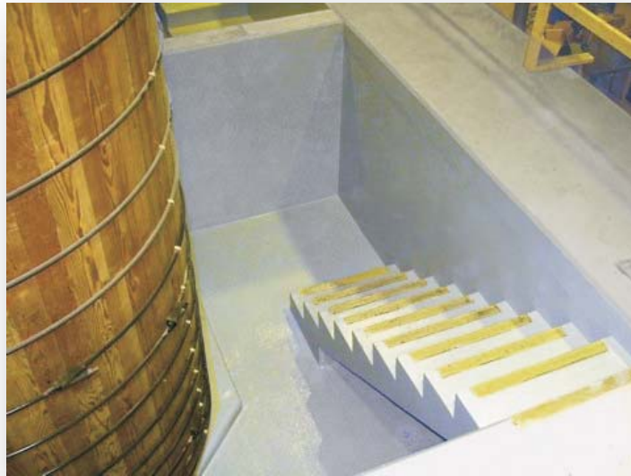
Completed containment lining in one chamber
