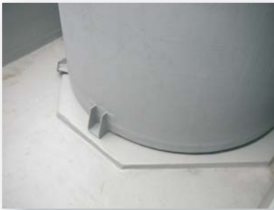
New tank and lining system
