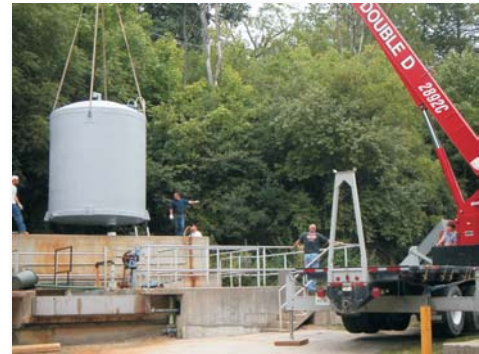
Placing the new tank
